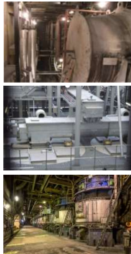
Figure 2. Biomass swirl burners, biomass feeding device and pulverizing chamber in Ferrybridge C Power Plant, UK (A, 2017) (a) Biomass Swirl Burner (b) Biomass Feeding System (c) Pulverizing Chamber
