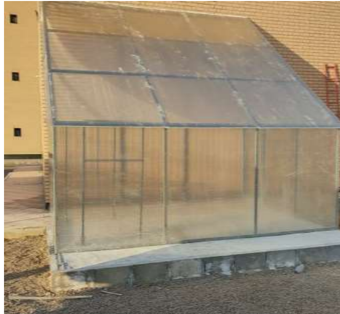
Figure 2. A view of the constructed prototype dryer
